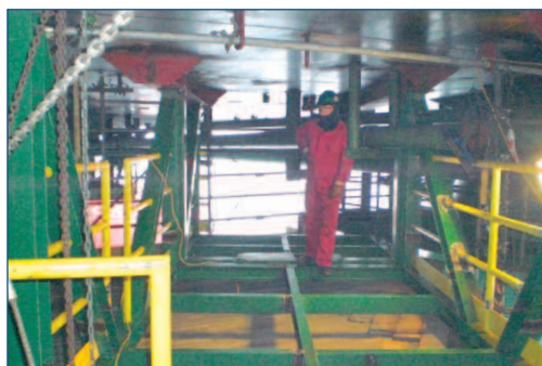
SUPPORT & ACCESS STEELWORK, prefabricated and installed for Ocean Rig's Leiv Erikson in preparation of the installation of ROPS arms
